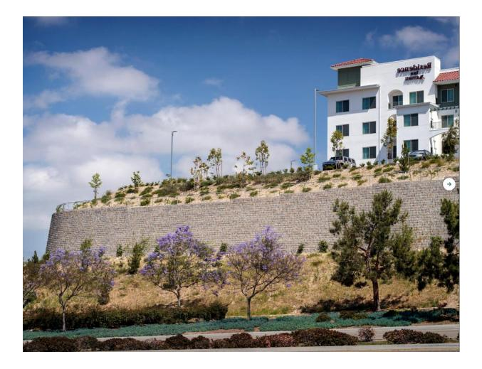
Belgard segmental retaining wall (SRW) products are produced by Oldcastle Architectural Products Group (APG) plants throughout North America and are manufactured in accordance with ASTM C1372 Standard Specification for Standard Specification for Dry-Cast Segmental Retaining Wall Units.
